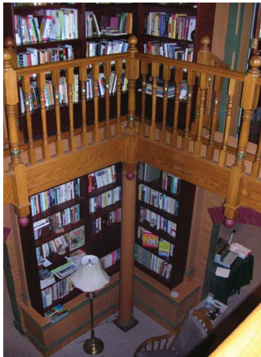
Keller removed the floor in the first-floor drawing room to create his two-story library.
